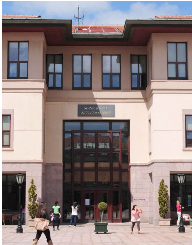
Top: View of Library from Maydan Bottom: Library - Main Entrance
