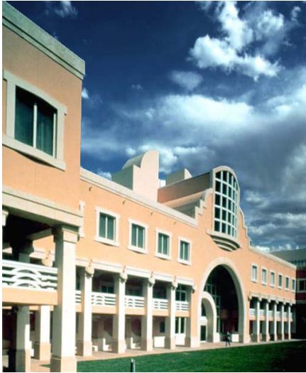
View from Courtyard
